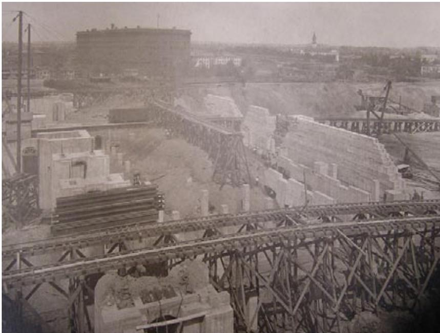
Conditions at the station in May 1905. The wall in the right center is the foundation for the wall to run between the headhouse and the concourse. Hopper cars dumped their dirt from the tracks running through the foreground, leading to the damage Thompson-Starrett protested. The building in the upper left is the Government Printing Office. (*Library of Congress*)
