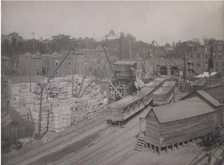
The New Jersey Avenue staging area. The structure in the middle of the picture is a concrete plant; the white area on the far right is laundry hanging from the back decks of the homes along the construction site. (*Library of Congress*)
