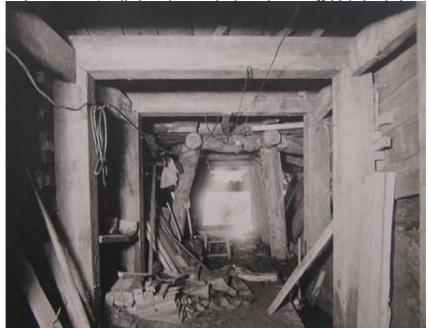
The top drift of the First Street tunnel, looking back to the southern entrance. In the foreground are the original square frames; closer to the light are the poles and crown bars
